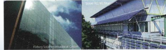
Photovoltaic panels as cladding
