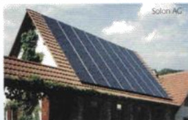
Photovoltaics installation on a house
